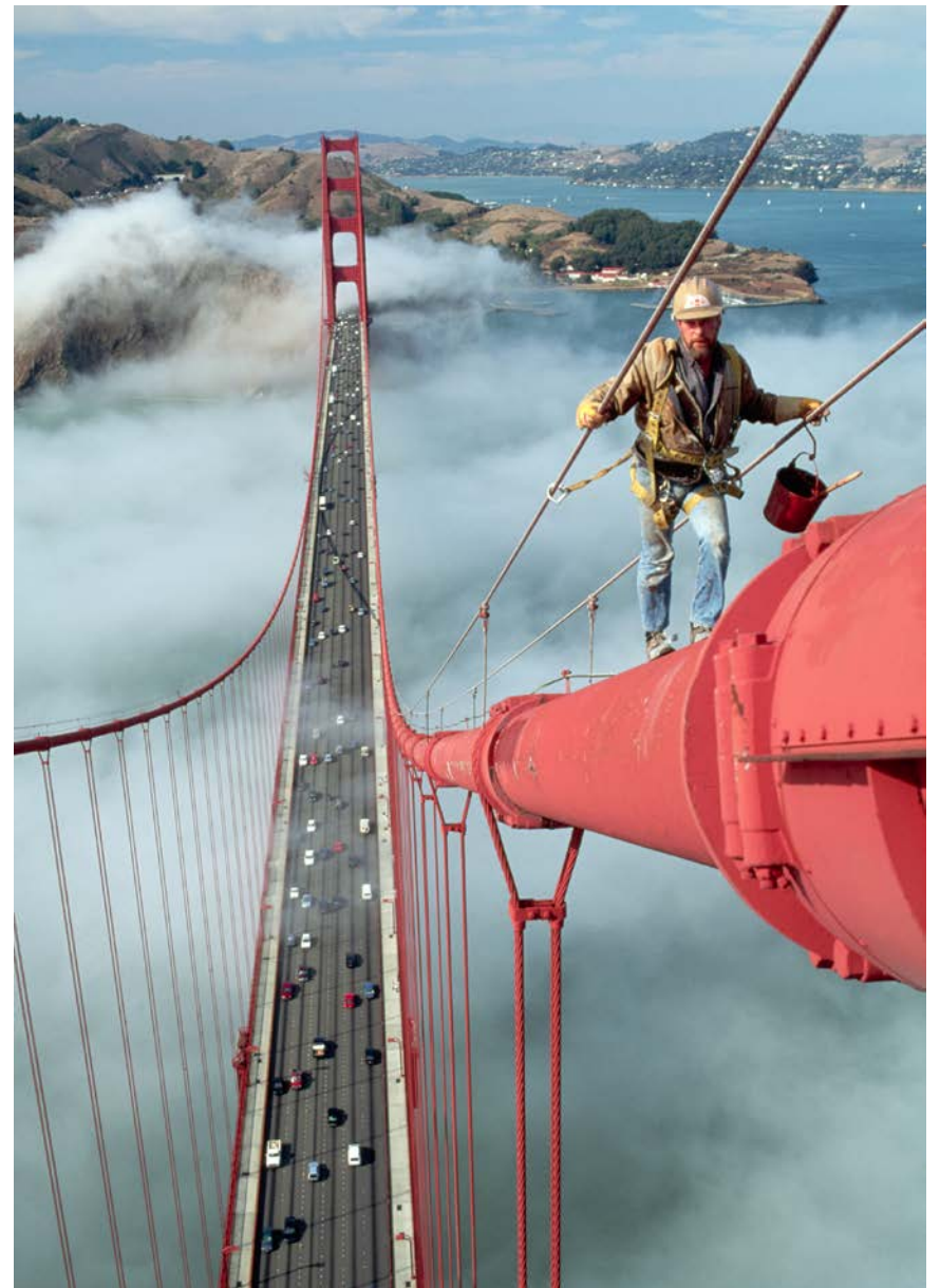
This painter works on bridges.
